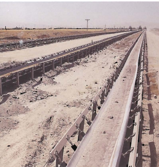
▲ Ash Conveying Belt / ST - 2000 / 1600 mm
