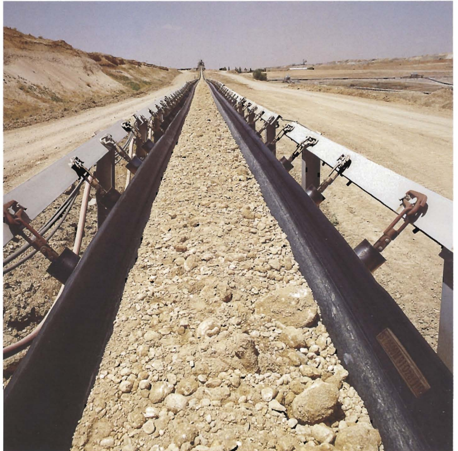
▲ Afşin/Elbistan Lignite Establishments Clay Belt 1800 mm/ST 2500
