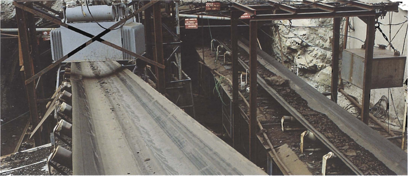
▼ Underground Coal Belt / ST - 1000 / 1200 mm
