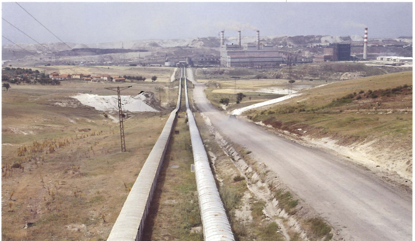
▲ Ash Conveying Belt / ST - 1800 / 1000 mm
